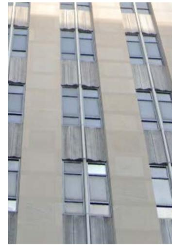
AFTER 12TH FLOOR BRIDGE REMOVAL, INSTALL SALVAGED FROM SOUTH TOWER, WINDOWS & ORNAMENTAL METAL PANELS TO MATCH EXISTING FACADE.
